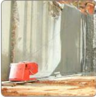
1. Granite Quarry Cutting
