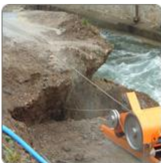
10. Concrete Cutting
